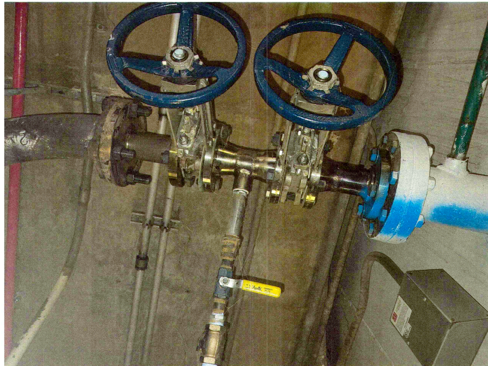
IMAGE OF ORIGINAL GATE VALVE ASSEMBLY
