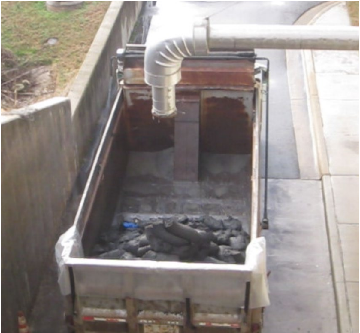
Figure 1. Sludge Chute
