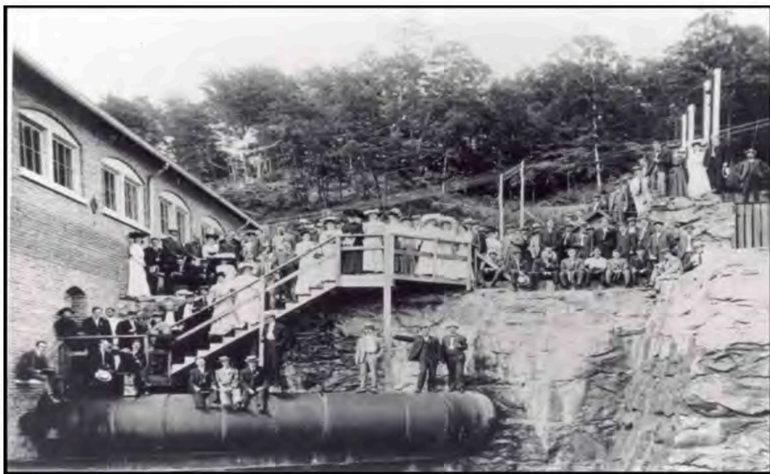
The Metropolitan Sewerage District of Buncombe County operates a hydroelectric facility on the French Broad River in Woodfin. The facility originally was built by W.T. Weaver in 1904 to provide electricity to Asheville, but MSD rehabbed it in 1984 to provide energy to treat the region’s wastewater. It can produce 2.5 megawatts of renewable energy. This photo is from the dedication ceremony in 1904. // Photo provided by MSD of Buncombe County
