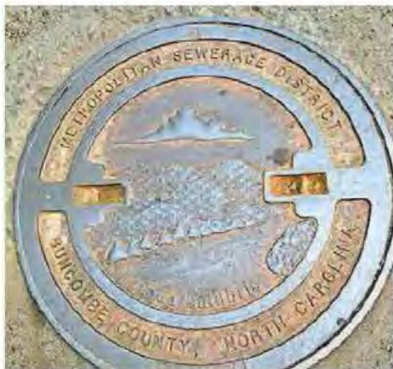
One of the Metropolitan Sewerage District of Buncombe County's current manhole covers is installed in a roadway in its sewer system.
