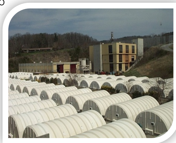
View of the MSD Treatment Facility
