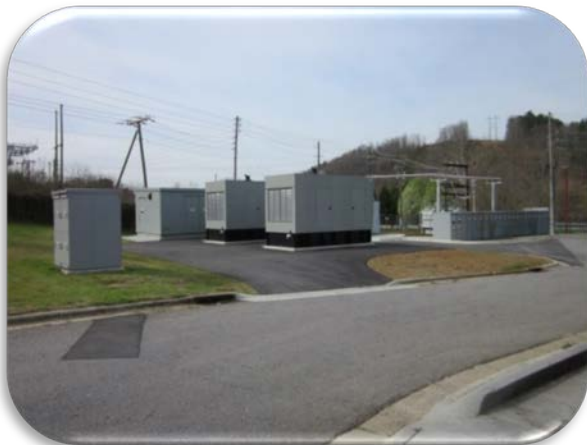
New Backup Generators and Controls, in Foreground
