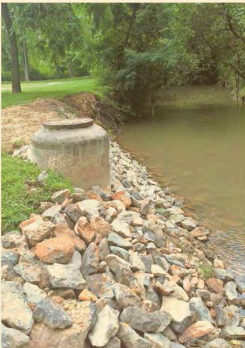
Manholes near creeks have to be raised out of the flood plain, according to MSD.
