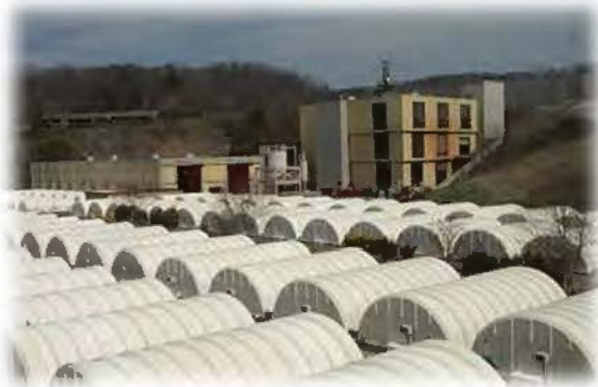
View of the MSD Treatment Facility
