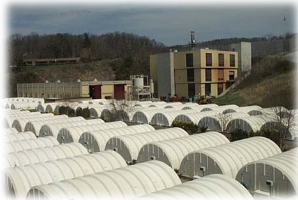
View of the MSD Treatment Facility
