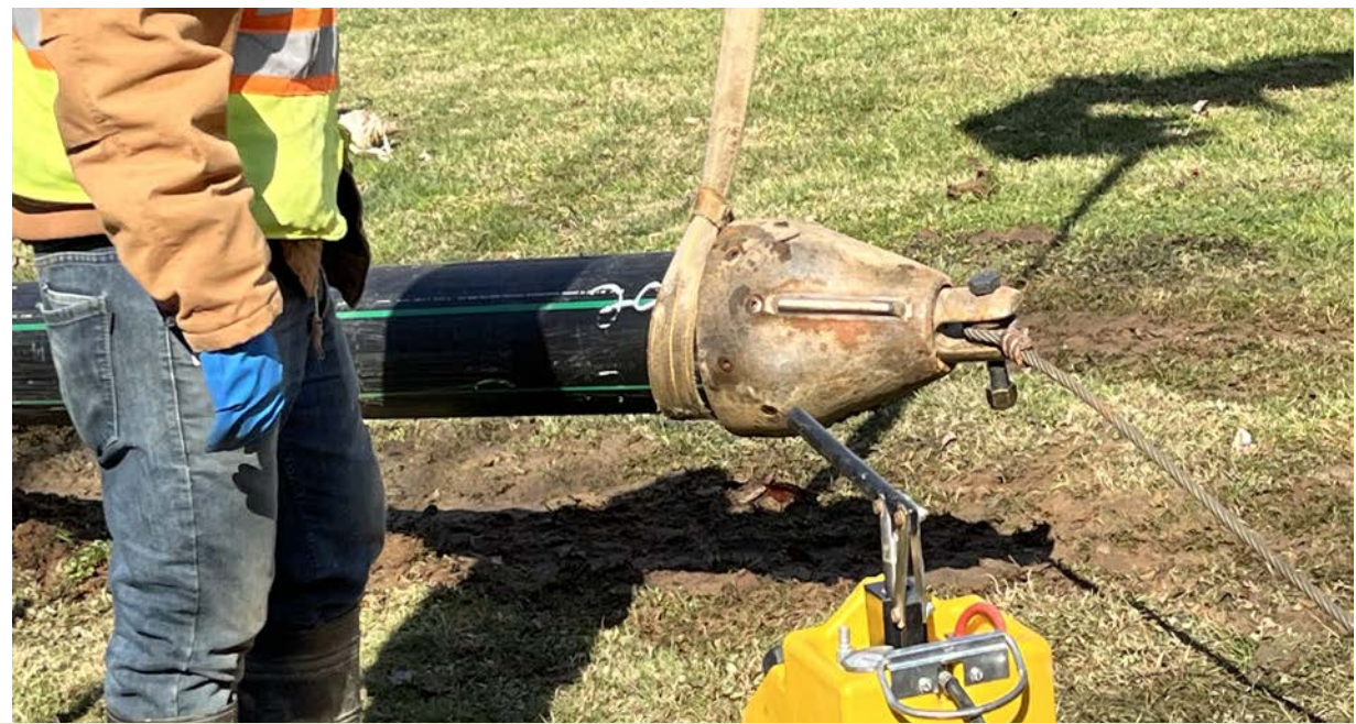
Pipe bursting bore pit (top left); bursting head and HDPE pipe (top right); winch machine (lower left); bursting head entering old manhole (lower right)
