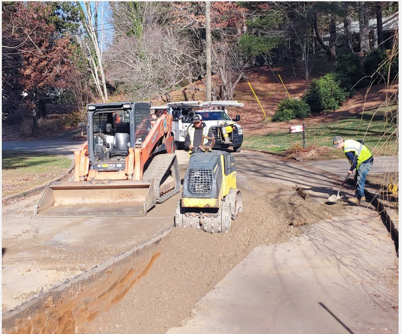
Trench compaction underway with Aggregate Base Course ("ABC")
