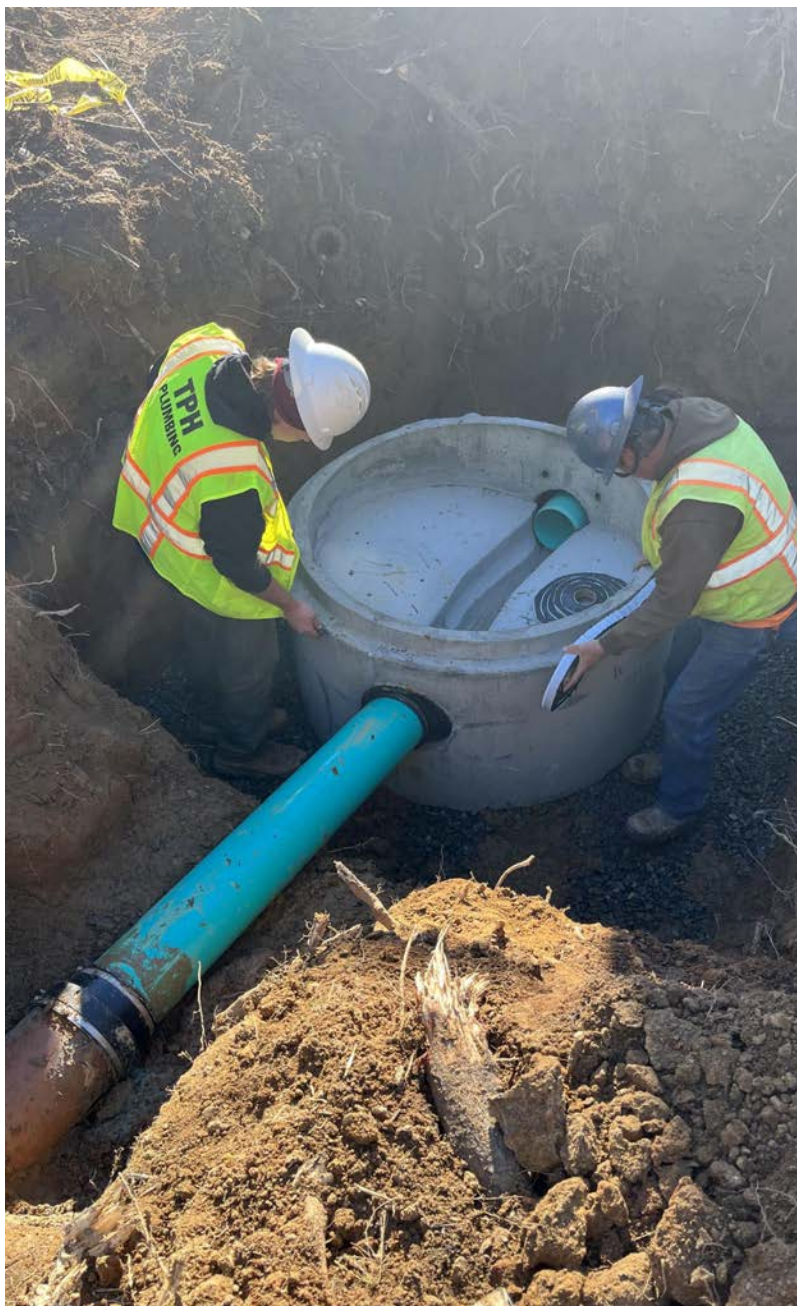
Installing butyl sealant on new manhole base
