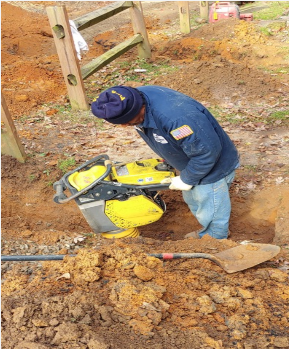
MSD's Elias Gutierrez compacting the backfill in a trench over the renewed sewer service line.
