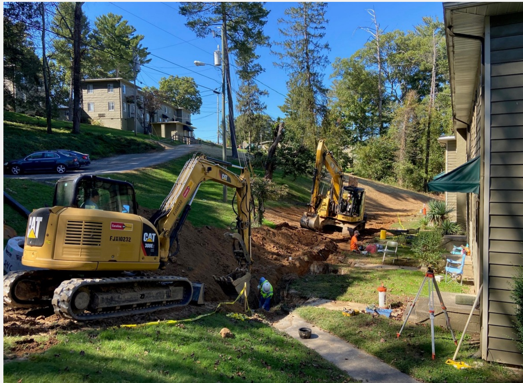
MSD crew working on mainline replacement behind apartment buildings on Conestee Street
