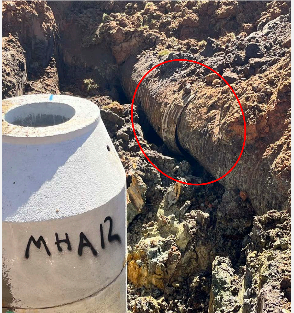
Deteriorated Corrugated Metal Pipe storm drains to be replaced by Huntley Construction following sewer line replacement
