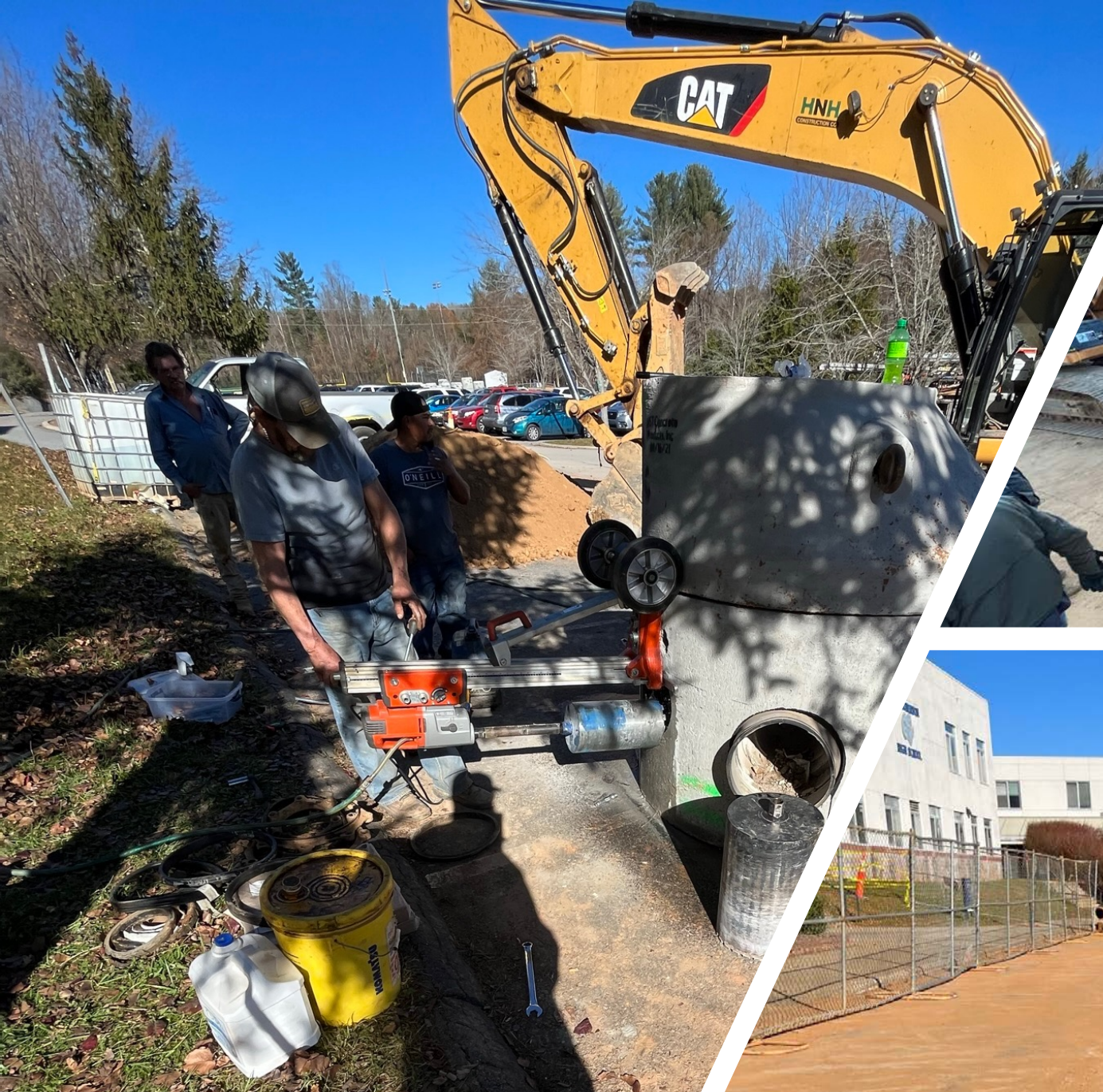
(Left) Coring manhole for new service line. (Right) Installing 8" main line adjacent to main school entrance
