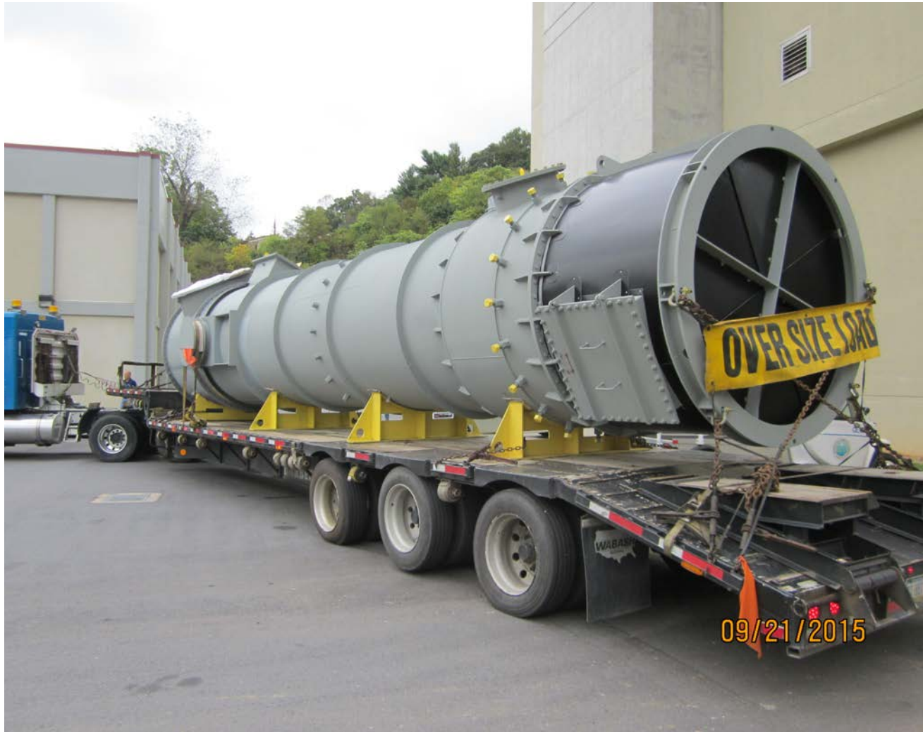
Replacing the heat exchanger in 2015. “Life expectancy 5-8 yrs” ( Industrial Furnace Company )
