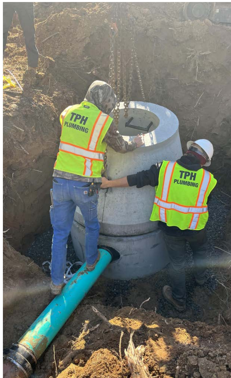
Installing manhole cone
