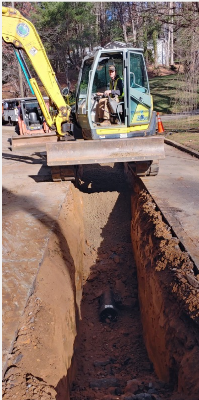
MSD's Matthew Ray installing 8-inch DIP
