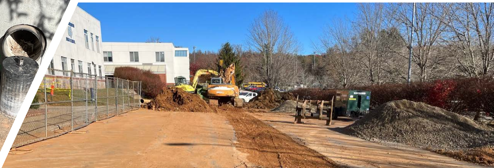
(Left) Coring manhole for new service line. (Right) Installing 8" main line adjacent to main school entrance
