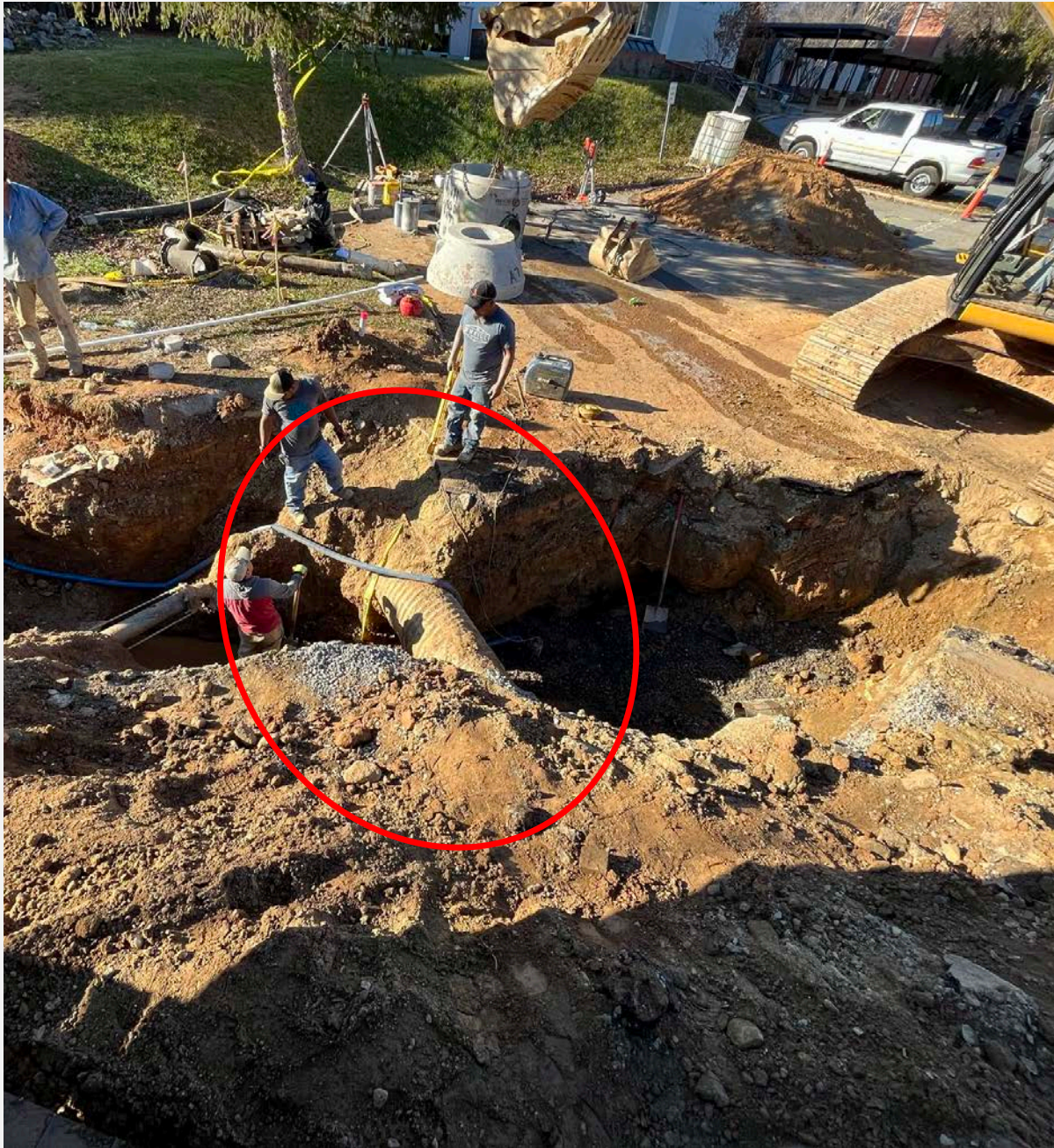
Deteriorated Corrugated Metal Pipe storm drains to be replaced by Huntley Construction following sewer line replacement
